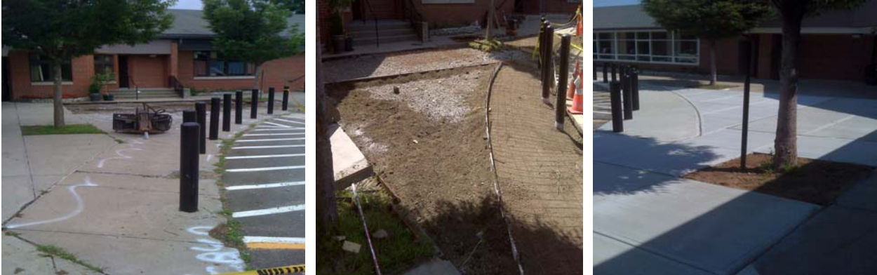
Side Walk Replacement
