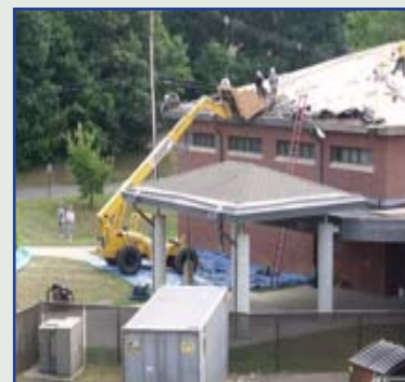
Roof Replacement at Lakes
